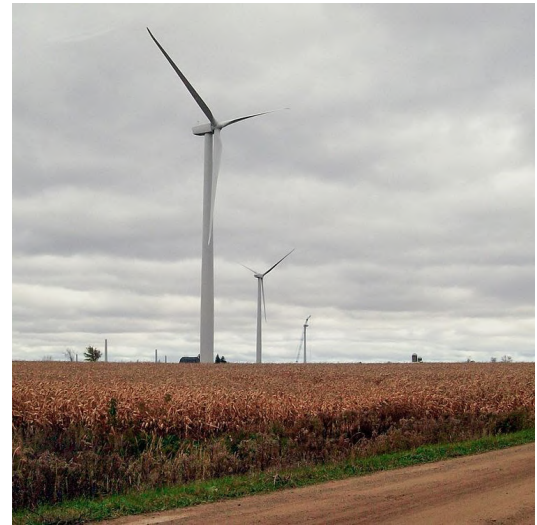
Wind Michigan 1 near Ubly, MI. Source: U.S. Department of Energy, 2015
